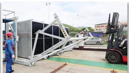
3. Use a crane or forklift to tilt the side wall onto the ground.
