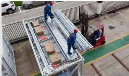
2. Lift the container onto the prepared ground, and take out the parts.
