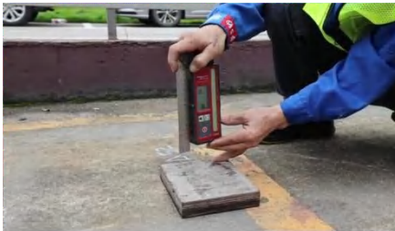
1. Leveling and ground preparation.
