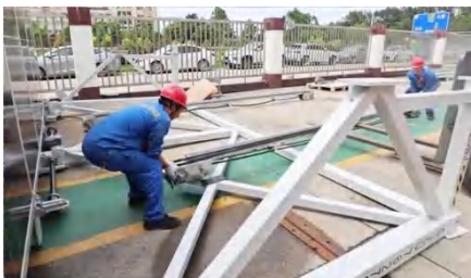
4. Install the tracks and the winch/motor.
