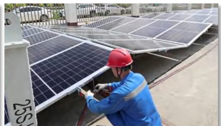
6. Connect the PV cable harness.
