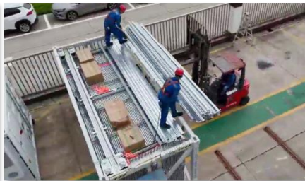
2. Lift the container onto the prepared ground, and take out the parts.
