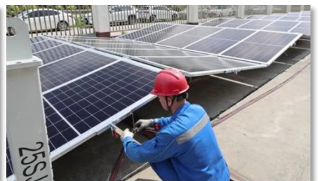
6. Connect the PV cable harness.
