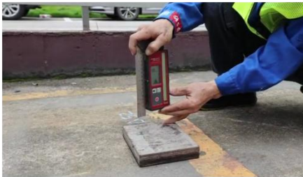
1. Leveling and ground preparation.
