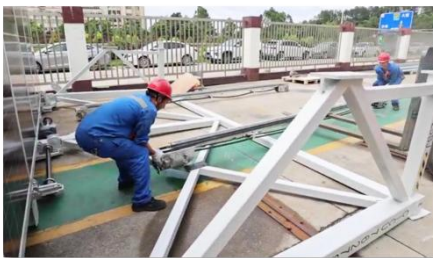
4. Install the tracks and the winch/motor.
