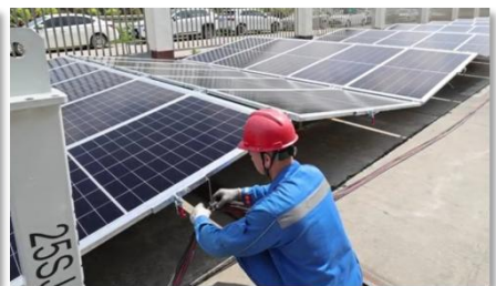
6. Connect the PV cable harness.
