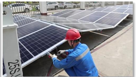
6. Connect the PV cable harness.
