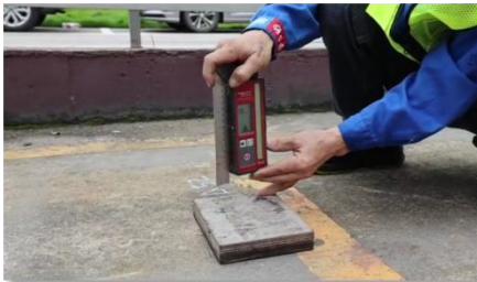
1. Leveling and ground preparation.
