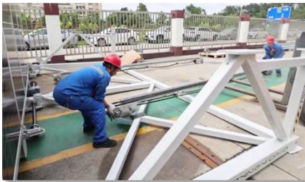
4. Install the tracks and the winch/motor.
